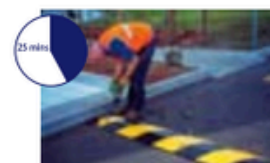
Insert & tighten fixings
