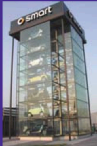
NUSSBAUM-TOWER XXL: The biggest of all smart-towers, in Hamburg, Germany. It holds 86 smart cars or 43 S-Class Mercedes, on an area of only 11 x 11m.
