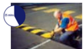
Trim rubber & clean site
