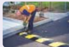
Insert & tighten fixings
