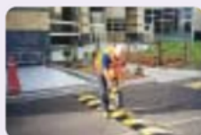
Drill holes for fixings
