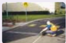
Lay down rubber base
